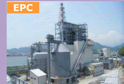
Biomass Power Plant
