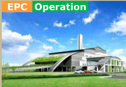
Waste to Energy Plant
