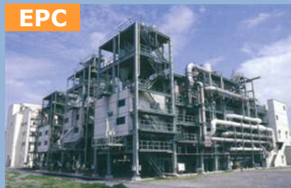
Sewage Sludge Incinerator
