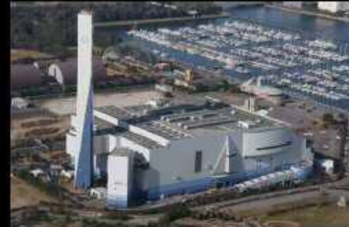
2010's Shin-Koto Incineration Plant
