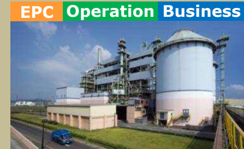
RDF Power Plant
