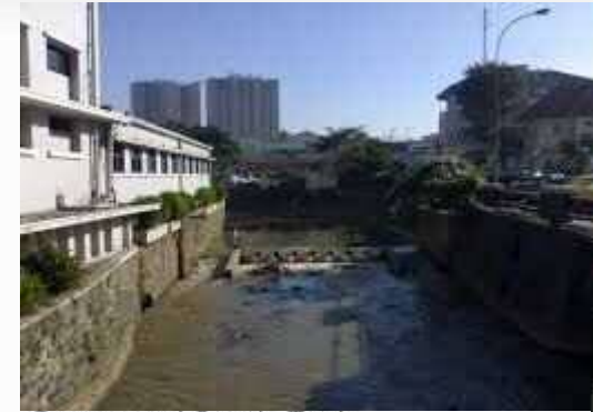
Communal Septic Tank
