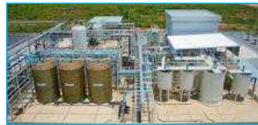
Wastewater treatment plant
