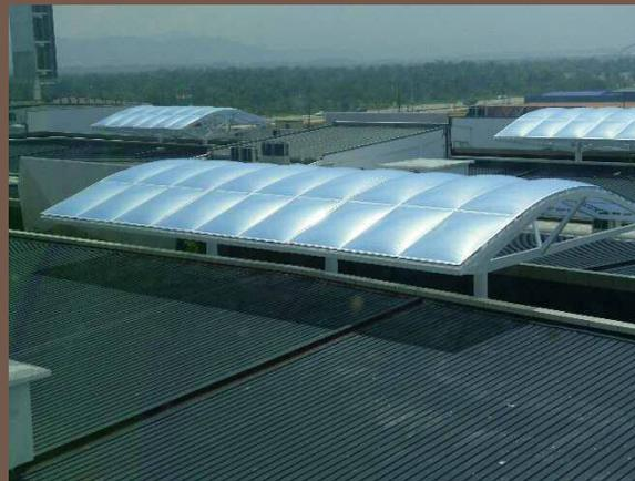
Plastic rooftop designed to trap heat inside from sunlight
