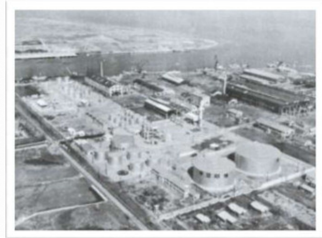
1955: TOA Oil's first refinery (6,000 barrels/day)
