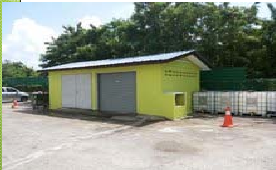
Taman Pelangi On-site Food Waste Processing Plant
