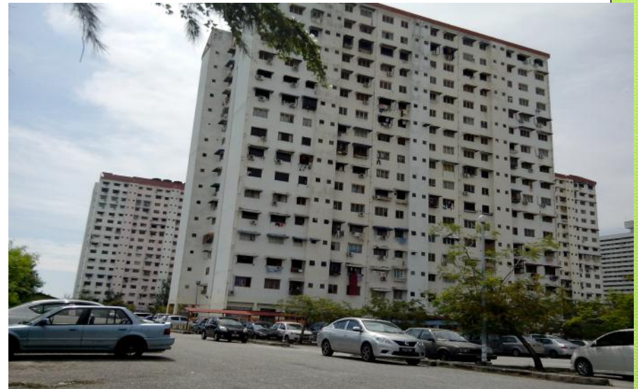
Taman Pelangi Medium Cost Apartments
