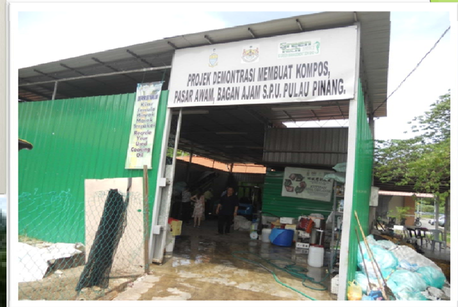
Bagan Ajam Wet Market Food Waste Processing Plant
