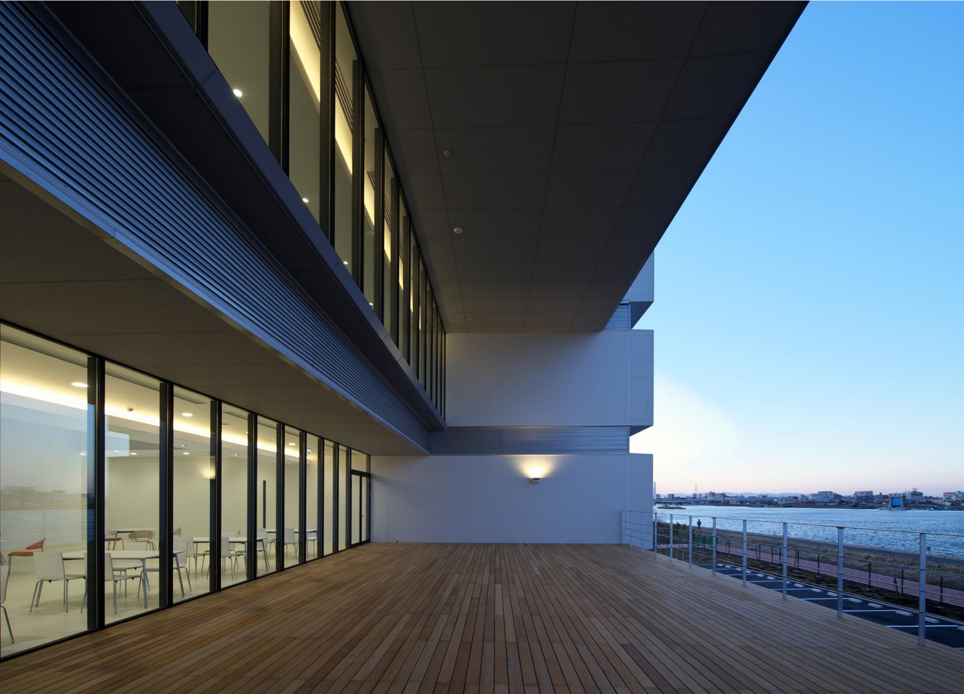
Second floor terrace
