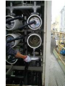
Membrane cartridge is exchanged for keeping its performance.
