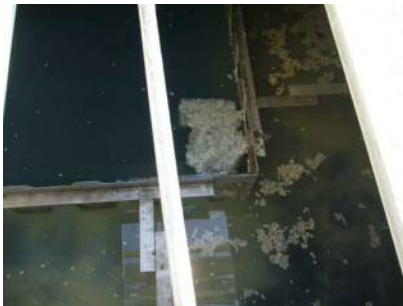
The wastewater include scum flow out from Sedimentation basin
