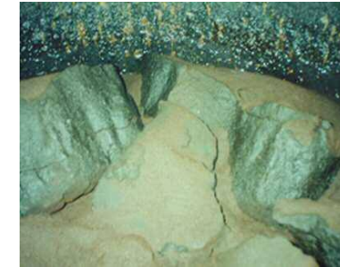
Filter exchange is required because the granular filter media is clogged and fixed by Suspended Solid.
