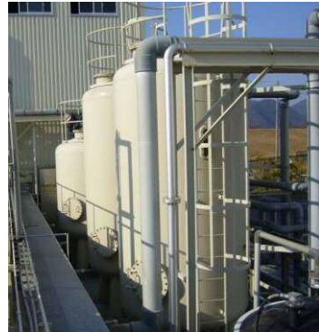
filtration machine of sand and activated carbon
