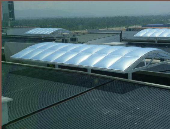
Plastic rooftop designed to trap heat inside from sunlight
