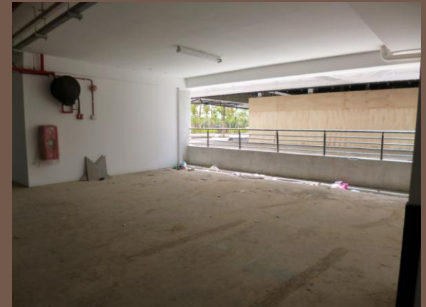
2 Electronic Vehicle Charging Station (charge Station) bays
