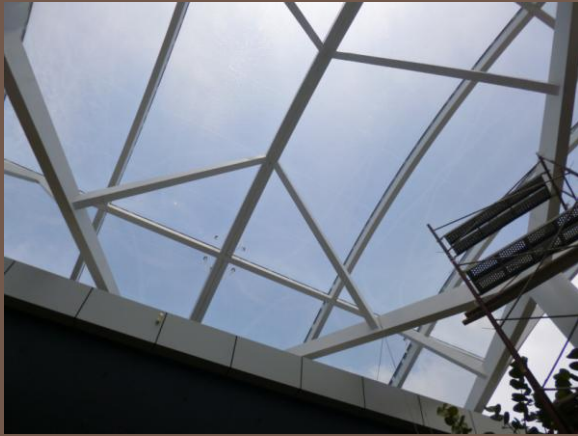
Glass Top Roof with Heat Insulation
