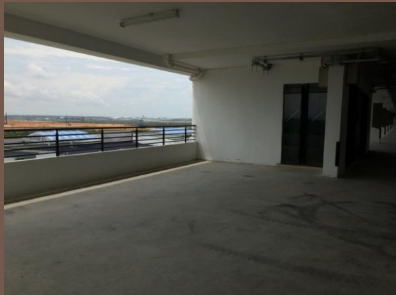
12 Disable Carpark Bays provided (Required 5 Disable Carpark Bays)
