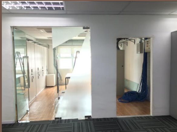
Control Room for Security purpose
