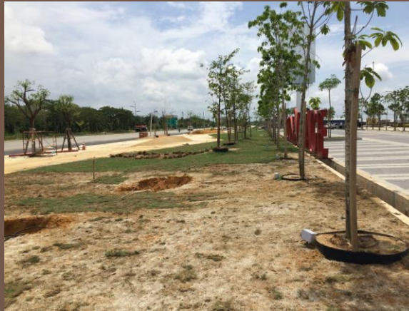
Soft & Hard Landscape construct on LRT/MRT reserved land
