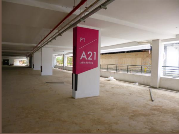
Ladies "Carparking Zone" on Level 1 of Multi-storey carpark building
