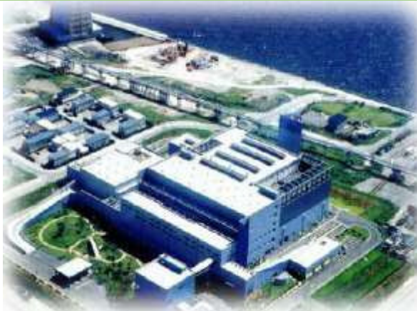
Ukishima Waste Treatment Center
