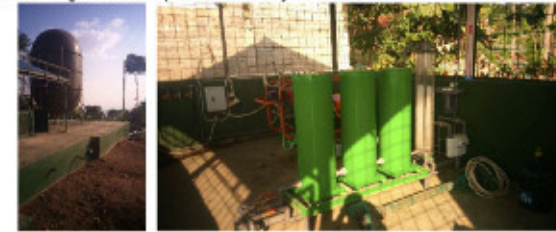
Installation of gas reactor to produce electricity for household needs
