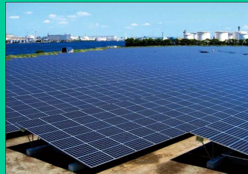
Ohgishima Solar Power Plant
