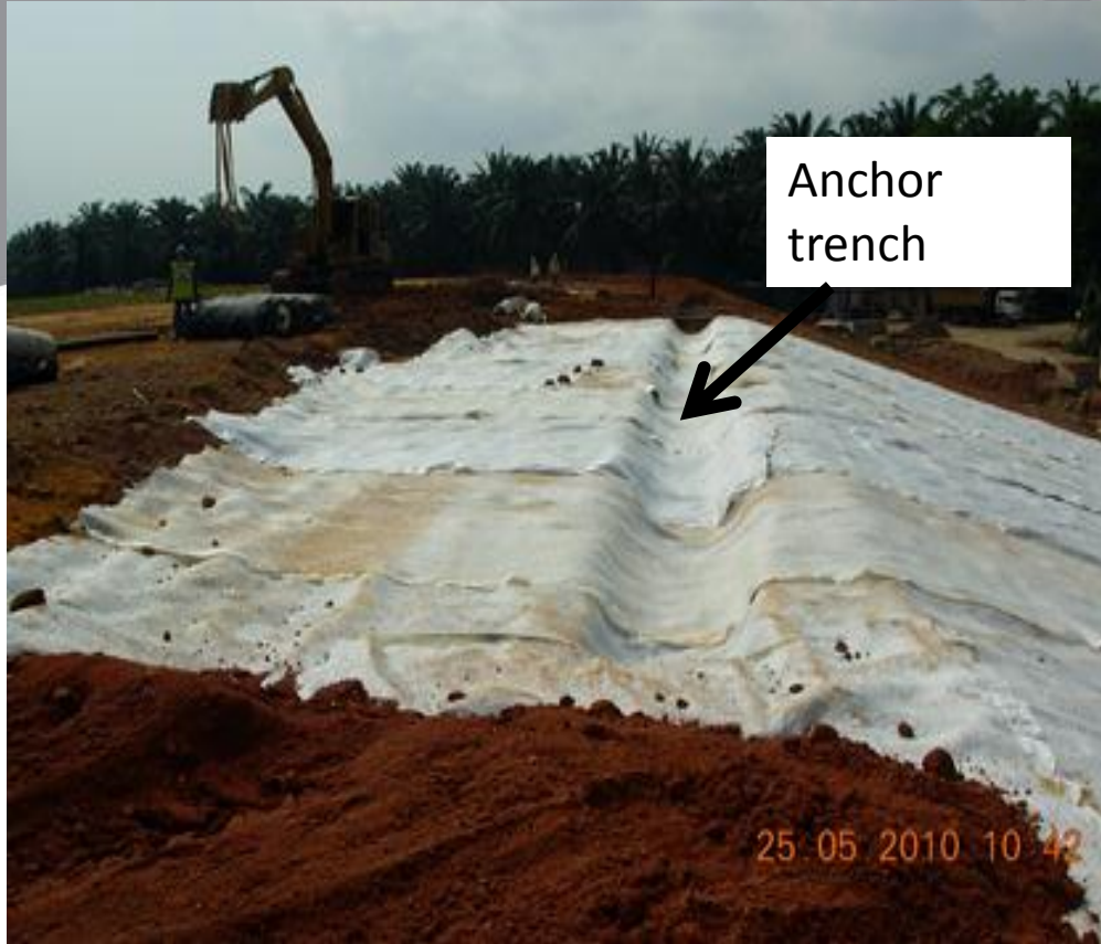
LAYING OF GEOSYNTHETIC CLAY LINER (GCL)
