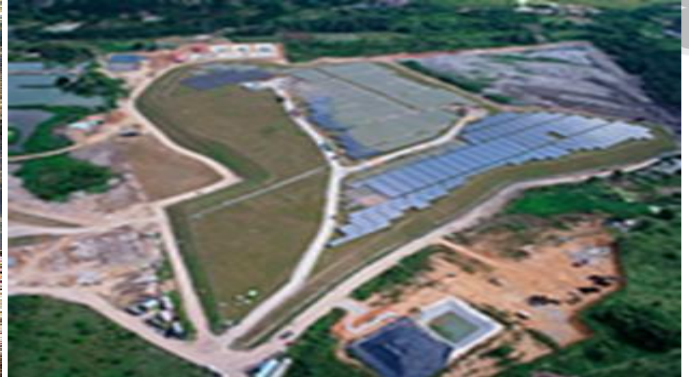
After safe closure
