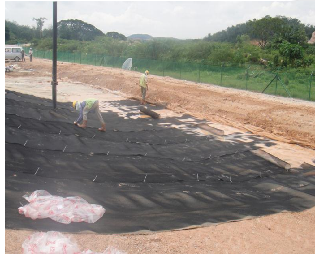
LAYING OF GEOSYNTHETIC DRAINAGE LINER ( GDL)
